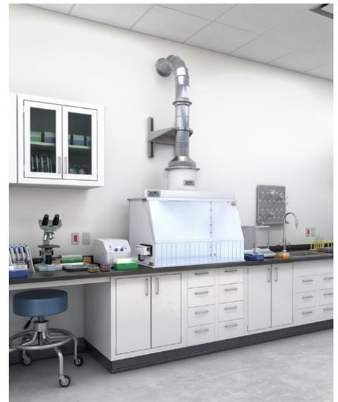
Inline Exhaust Fan attached to Ducted Fume Hood in a lab setting
