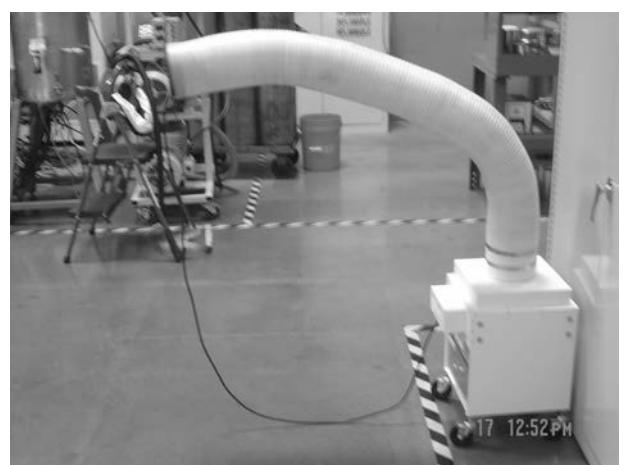
**FIGURE 1.** Photo of Local Exhaust Ventilation (LEV) used during reactor cleanout procedure
